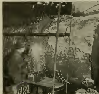
FIG. 2.—BOILER REPAIRING BY ARC WELDER.
